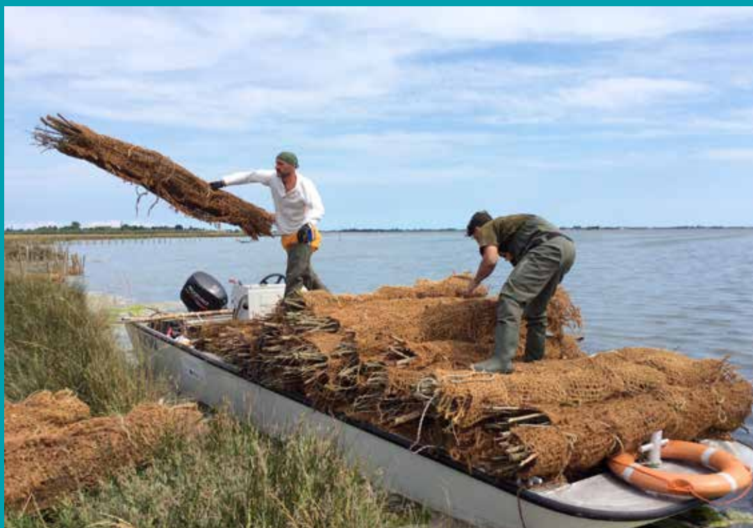
Fascines ready to use are unloaded on a salt marsh
