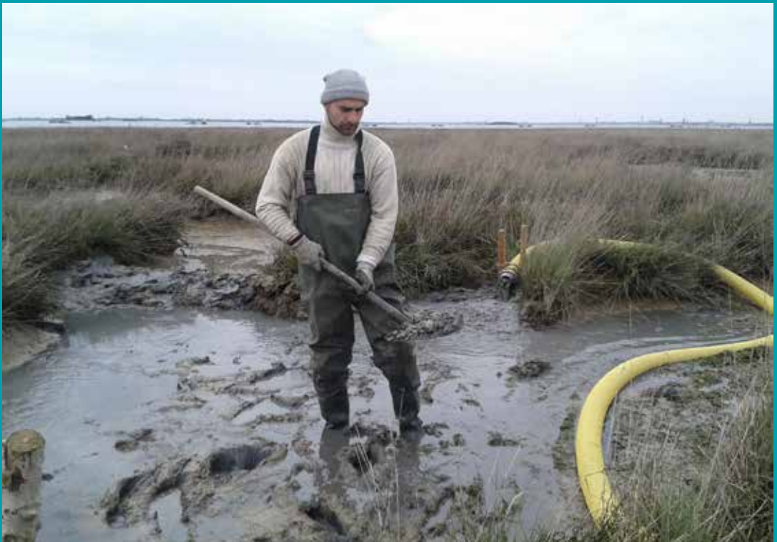
Sediment pumped behind the fascines to restore an eroded portion of salt marsh
