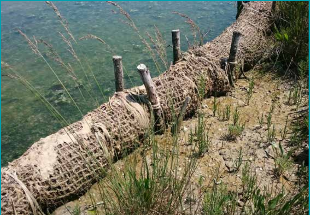
The mud nourished behind the fascines is quickly colonized by salt marsh plants
