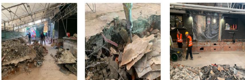
Figure 2. Strip out demolition applied in the case study.
