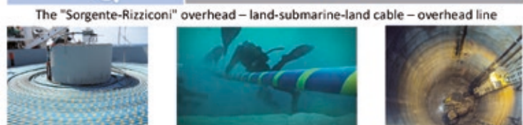
From left: Cable drum in the cable laying ship Giulio Verne; an installation phase of the submarine laying; an impressive view into the vertical tunnel
